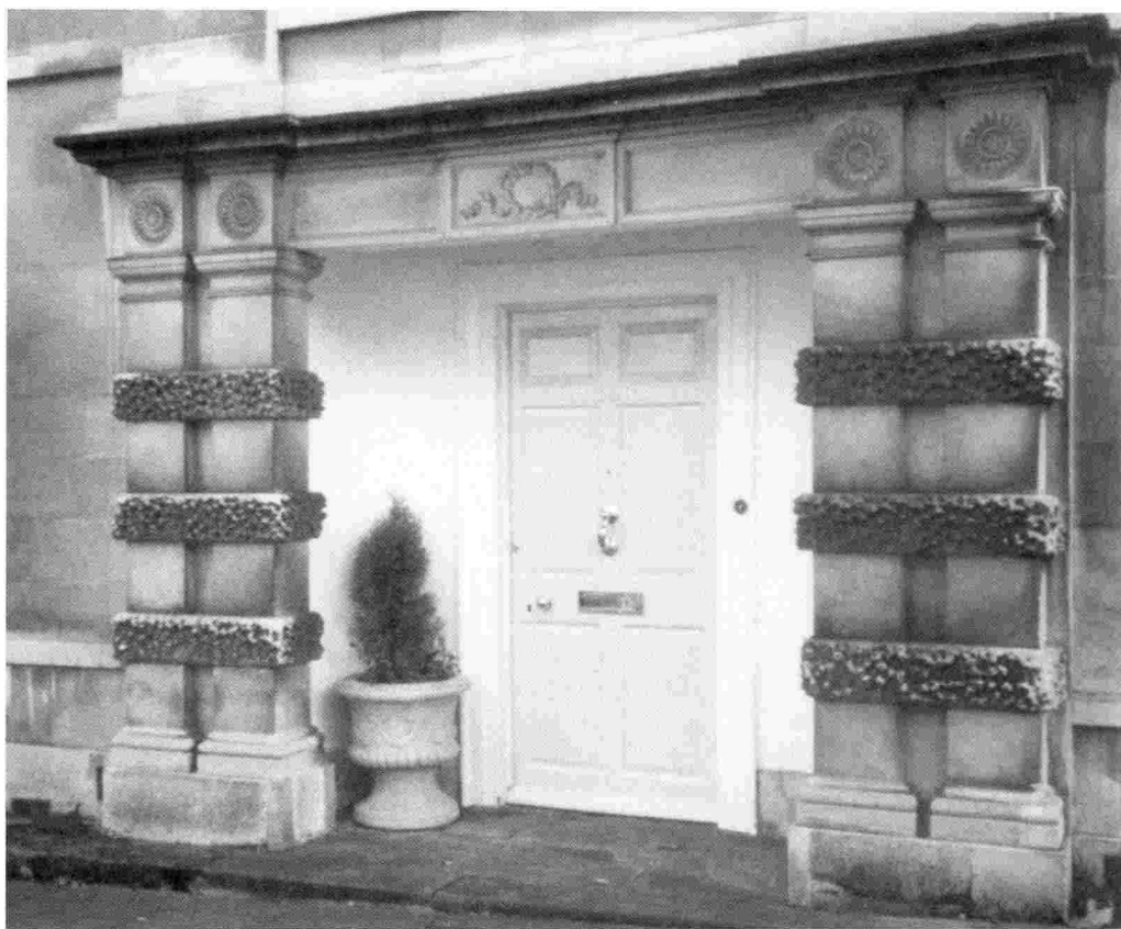
FIG. 136 – No. 5 Honey Hill, Bury St Edmunds: detail of door surround.
